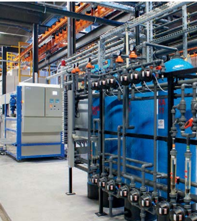
Decentralized, process-integrated wastewater treatment plant and water recycling for the automotive industry.
